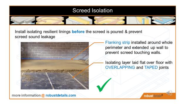
The resilient system, comprising of the resilient layer and flanking edge strips, must be fully installed and secured before the screed goes down
