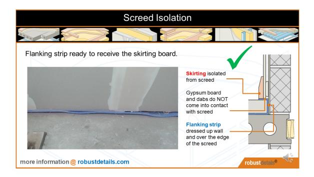
Resilient flanking strip must be dressed up the edge and over top of floating screed. This will isolate the screed from wall linings; and when the skirting board is affixed to the wall, it will sit above the flanking strip – and not on the screed.
