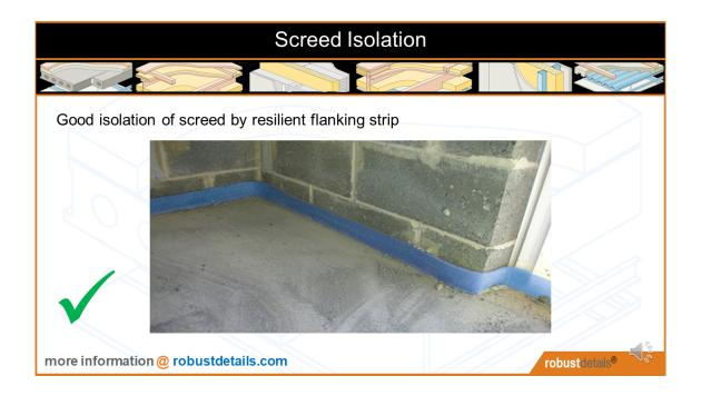
Flanking strip properly installed around the perimeter – just remember to fold it down before applying the wall finishes.
