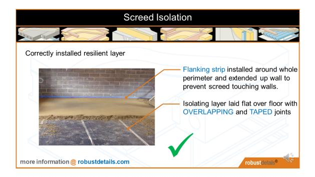
This is a photograph shows correctly installed resilient layer remaining firmly in place during application of the screed.
