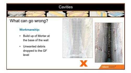
As well as mortar collecting on wall ties, a much more significant issue is allowing it to accumulate at the base of the wall, as it creates an acoustic bridge for the whole length of the wall.
