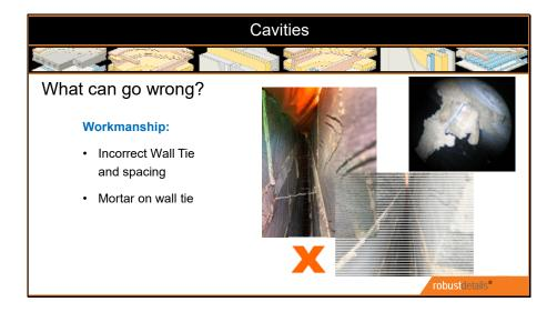
We've just spoken about the importance of NOT using ties that are so long they have to be put in diagonally;
