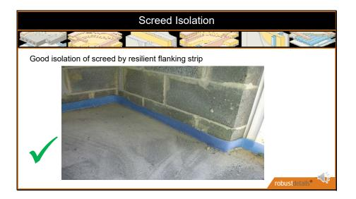
Flanking strip properly installed around the perimeter – just remember to fold it down before applying the wall finishes.
